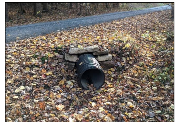
Properly installed smooth-bore plastic pipes are self-cleaning.
