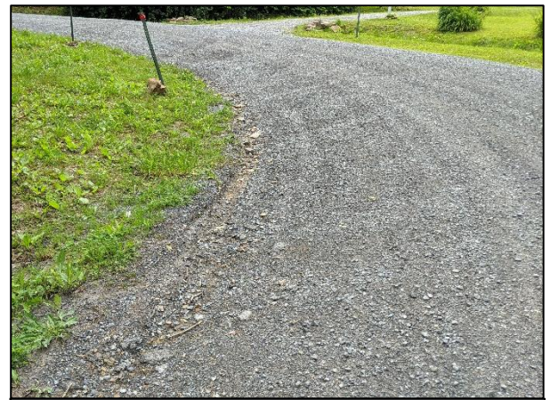
“Wash boarding” is one sign that it is time to grade an unpaved road.
