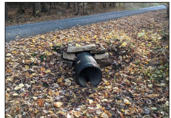
Properly installed smooth-bore plastic pipes are self-cleaning.
